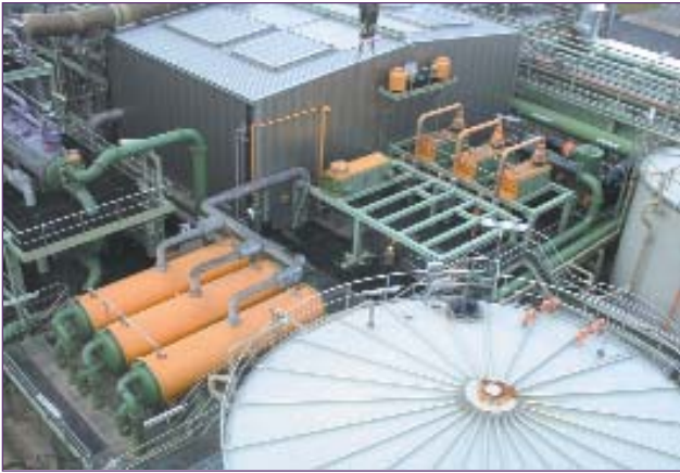
Figure 5. S&T condensers are shown on the lower left, and three welded block plate condensers are shown on the top right. Despite their small size, the block condensers have 50% greater capacity than the S&T units.
