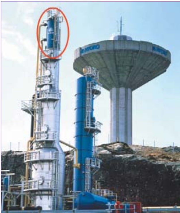
Figure 2. In this installation, the column mounted spiral condenser is on a stripping column.
