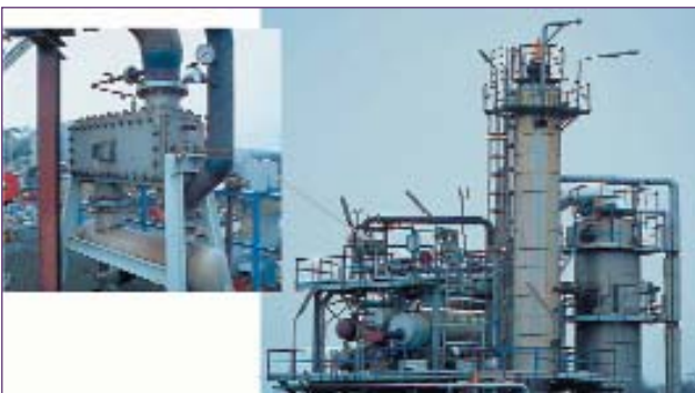
Figure 3. One of two welded block plate condensers on the vacuum column. The pressure is approximately 0.3 bara.
