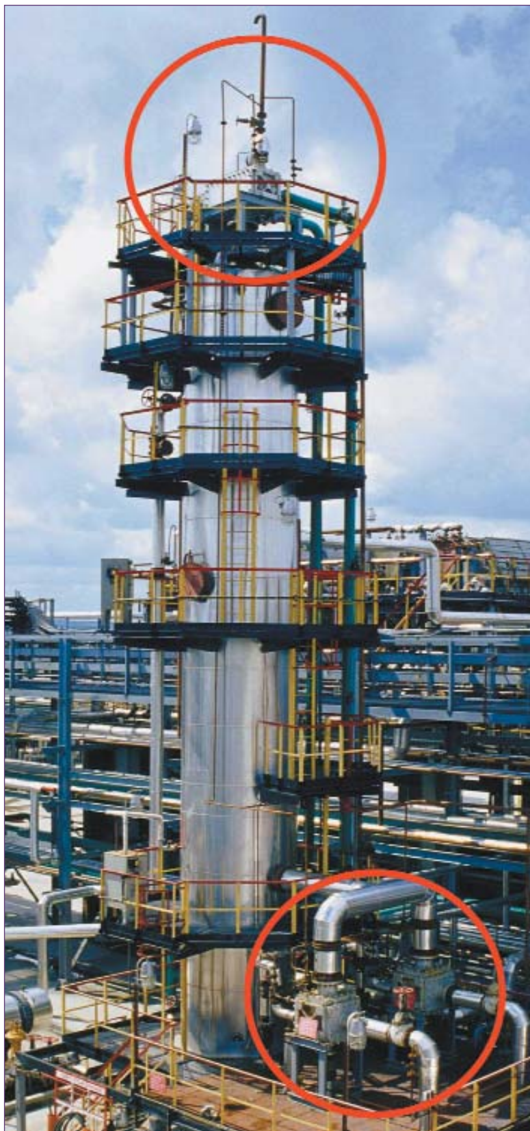
Figure 4. An absorption/stripping system used to clean a C1-C4 gas coming from the cracker of H 2 S. This column has a welded block condenser designed as a top mounted partial reflux condenser. There is also a welded block plate reboiler installed where a 15% MEA solution is evaporated at 127 °C using steam at 170 °C.
