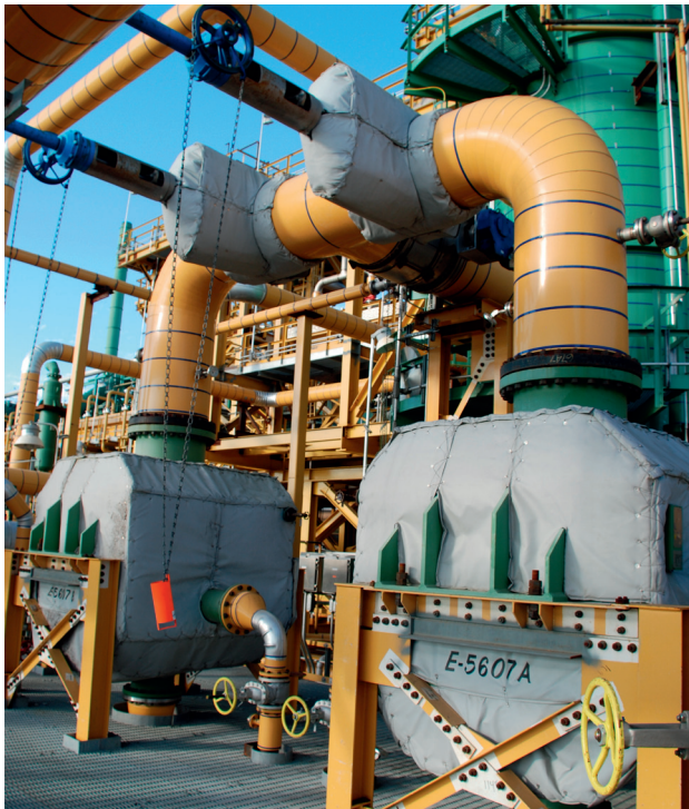
Two compact CPX 120 reboilers efficiently add heat to a CANSOLV® lean amine stripping tower. PHOTO: Jim Hill.
