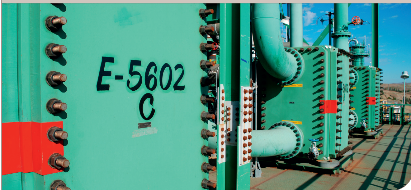
Three Compabloc CPX 120 heat exchangers ensure environmental compliance in a BELCO® flue gas scrubber. PHOTO: Jim Hill.
